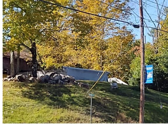
Foundation from Moultonville Road
