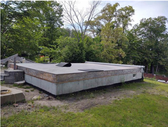
2019 30'x20' poured concrete Foundation
