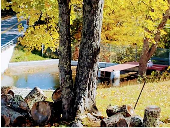
swimming hole at Dam
