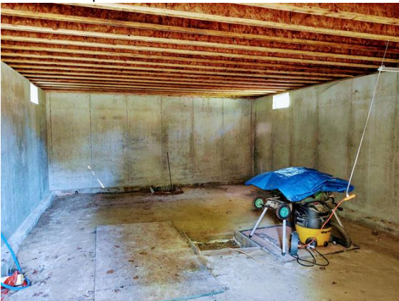
full Basement, with floor joists above
