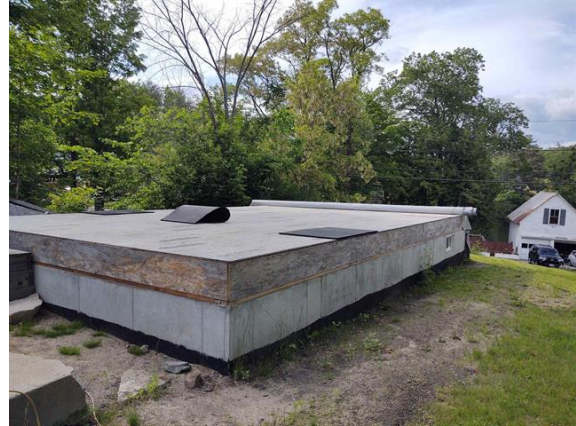
2019 poured concrete foundation (30'x20'), capped
