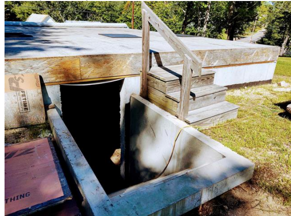
installed stairwell, to Full Basement
