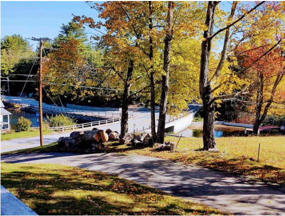
from 2019 Foundation, towards Mill Pond & Dam
