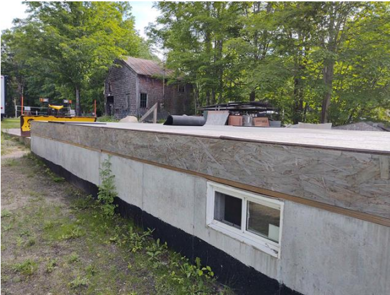
...with full basement under
